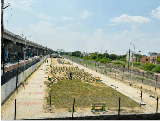
Current Photo of ongoing work
