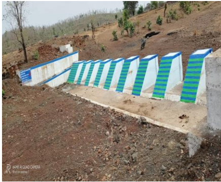
Stop Dam, Village: Ranidhar,
