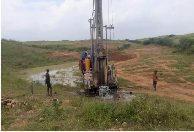
Installation of Bore well in pastureland
