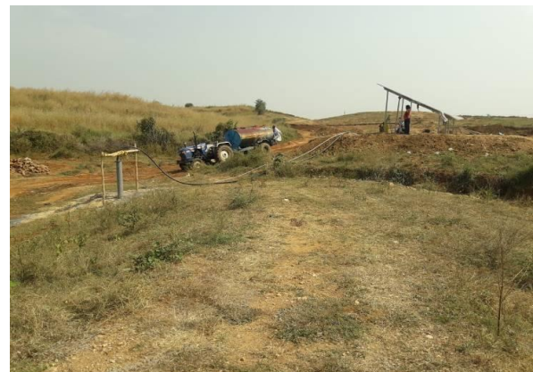
Work done of Solar pump
