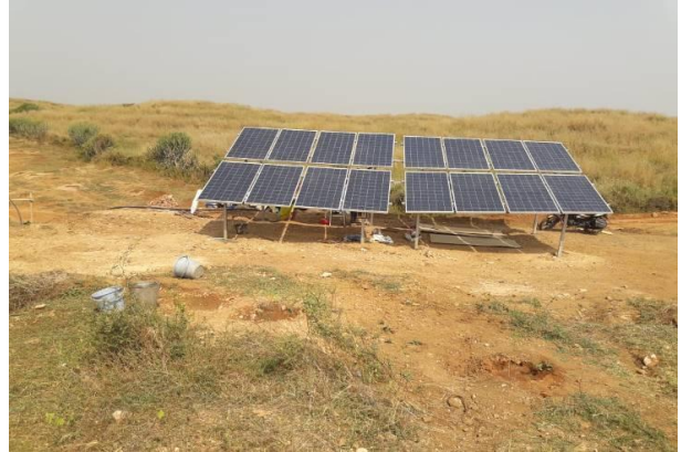
Installation of Solar pump in pastureland
